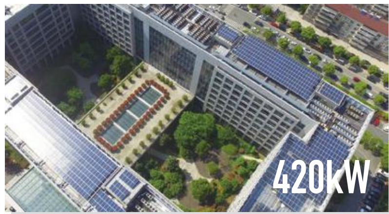
Project Type: Commercial Rooftop Location: China / Changzhou Commission Date: 2017-5 Product: SRP-265-6PB
