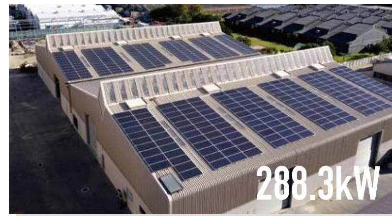
Project Type: Commercial Rooftop Location: South Africa / Cape Town Commission Date: 2018-3 Product: SRP-320-6PA
